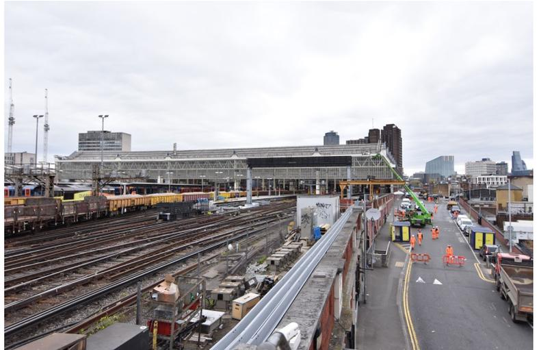
The new signalling gantry now extends over platforms 1-8, and has been carried out ahead of work to extend platforms 1-4, which Network Rail will undertake during a three-and-a-half week part-closure of Waterloo station in August 2017.
